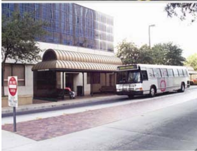
Provisions for transit travelers with buildings oriented to transit in Tampa.
