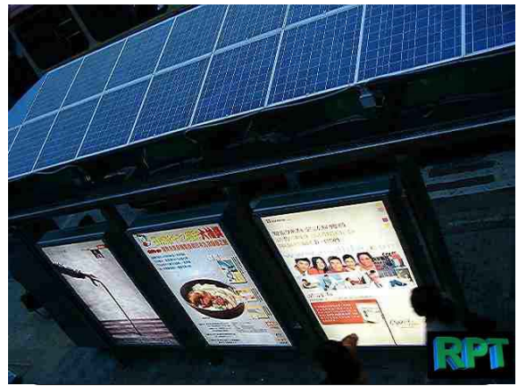
The solar powered bus shelter illuminates its information systems and advertising panels with power generated by photovoltaic panels, independent of the electricity grid.
