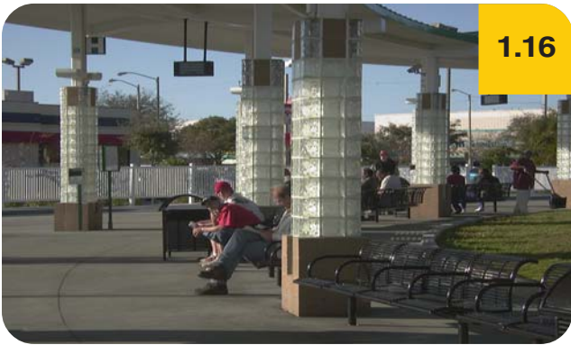
Divided bus bench seating at an intermodal bus passenger facility in downtown St. Petersburg, FL.
