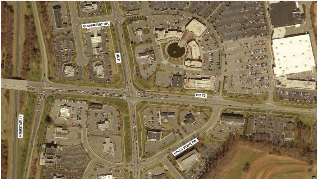
FIGURE 4 I-77 and NC 73 Interchange Vicinity
