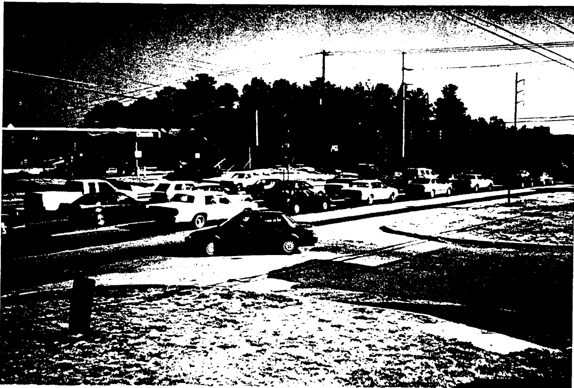
Figure 1 - Driveway Close To Intersections Invite Hazardous Left Turns
