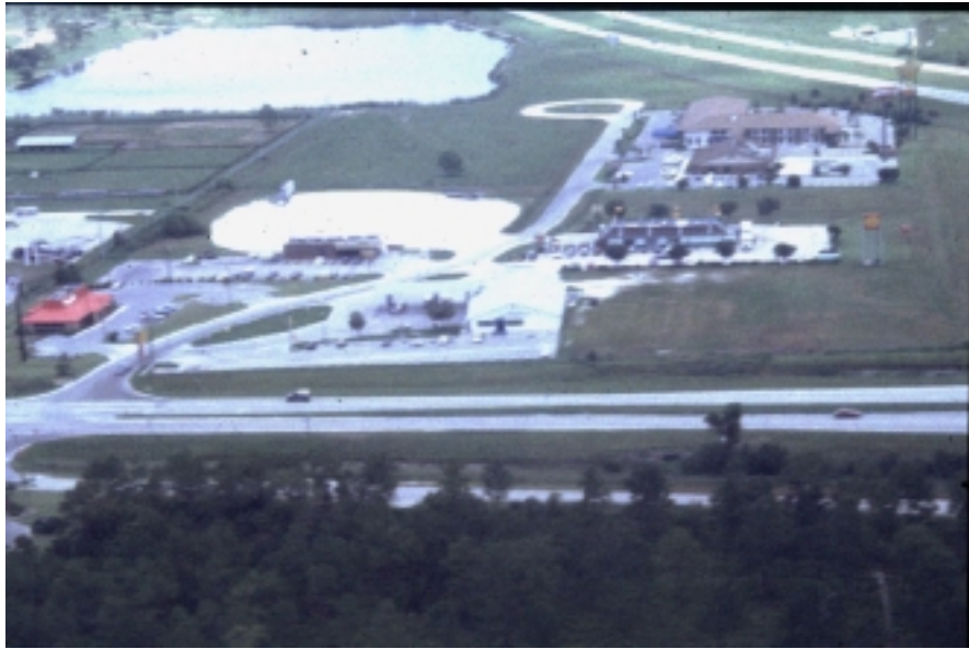
Figure 1 Access Road in Punta Gorda, Florida
