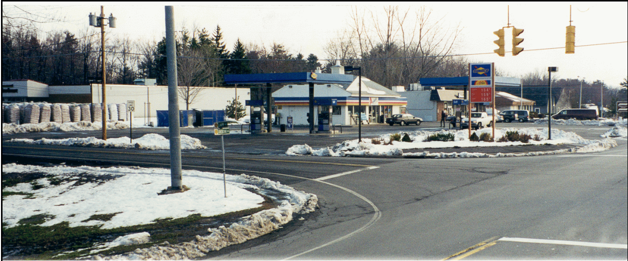
Figure 3: Outreach is Most Effective in the Local Context – In this case, a number of accidents between vehicles turning right and vehicles exiting the facing driveway served to illustrate the problems associated with inadequate corner clearance.
