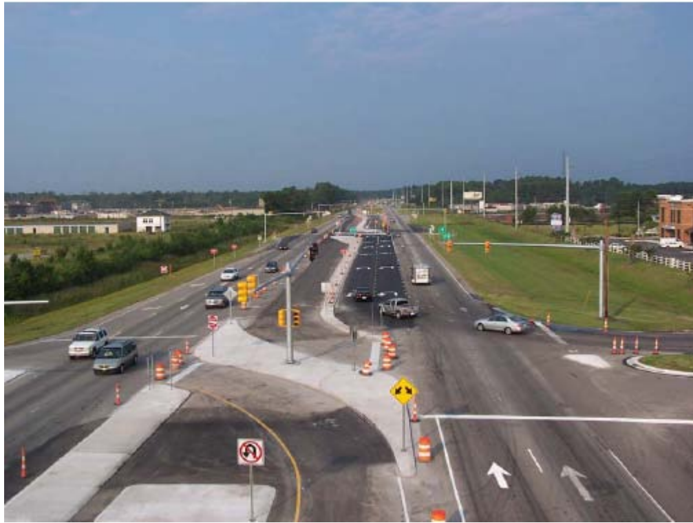
Figure 3. US-17 superstreet late in construction phase. Photo courtesy of the NCDOT.
