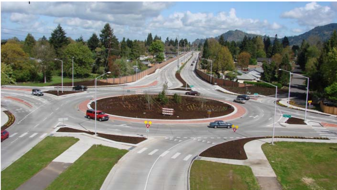
Figure 16: MLK Boulevard - Springfield, OR (Source: Brian Barnett, City of Springfield Traffic Department)
