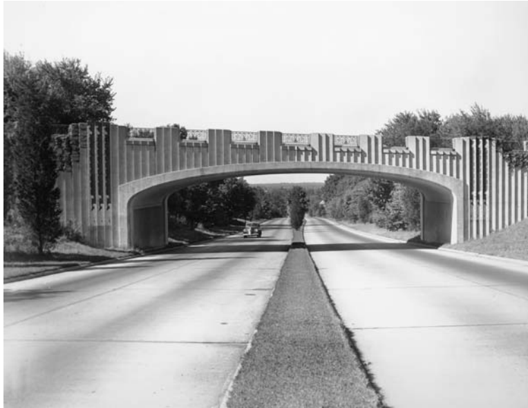
The Merritt Parkway featured 69 showpiece bridges designed to frame the view. This is the North Avenue Bridge in Westport.
