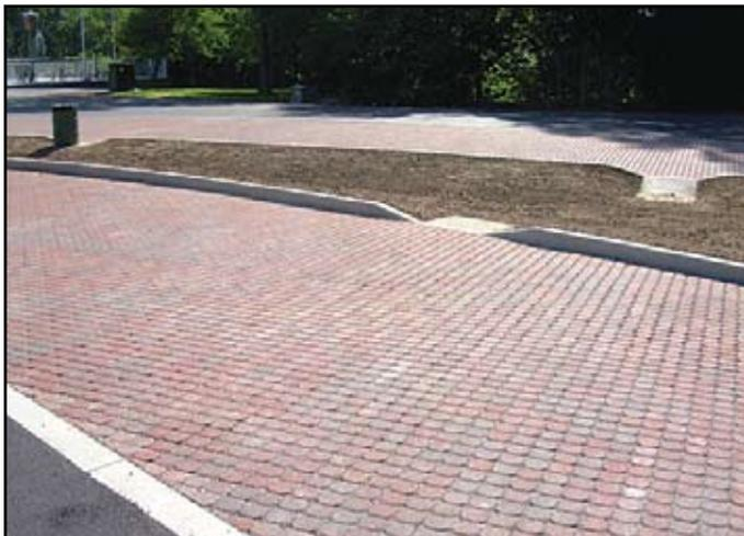
**Figure 3.20** | Pervious paver block parking lot.
