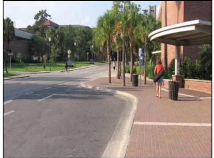
**Figure 5.5** | Bus bays allow buses to safely re-enter traffic.
