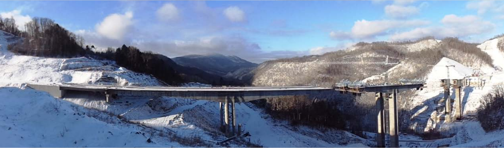
The Route 460 Connector Bridge in VDOT's Bristol District (Buchanan County) was recently ranked as the top bridge project in North America by Roads and Bridges Magazine . (photo credit: Tom Mackey, AMT)
