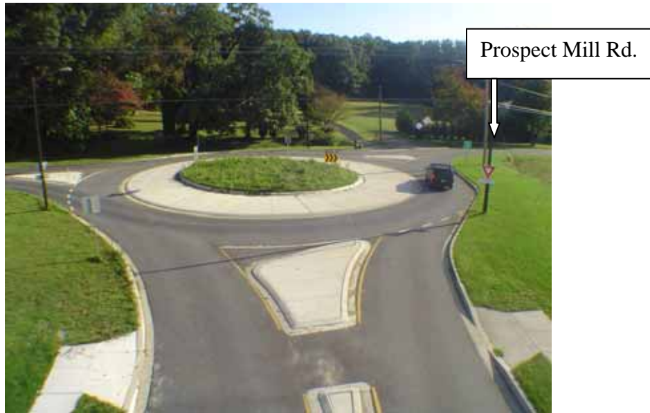
Prospect Mill Road/Wagner Road Roundabout
