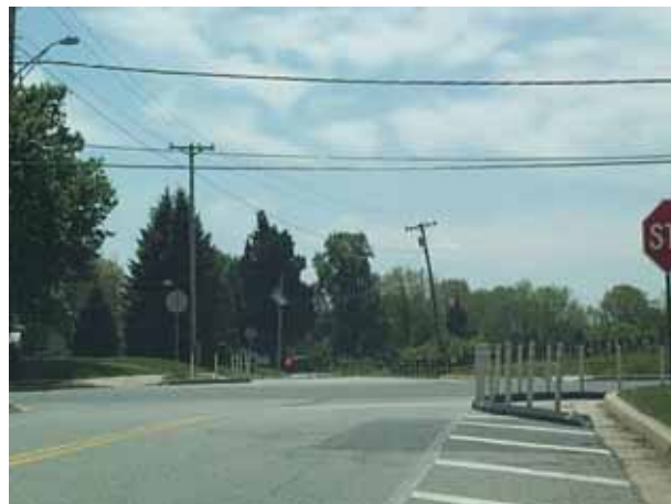
Temporary curbing on side road approaches
