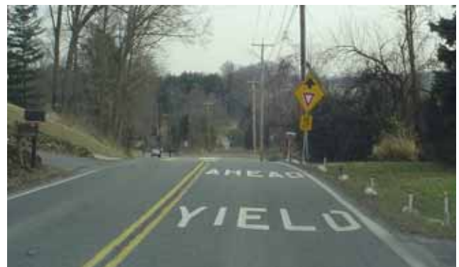
Advanced roadway markings and signing
