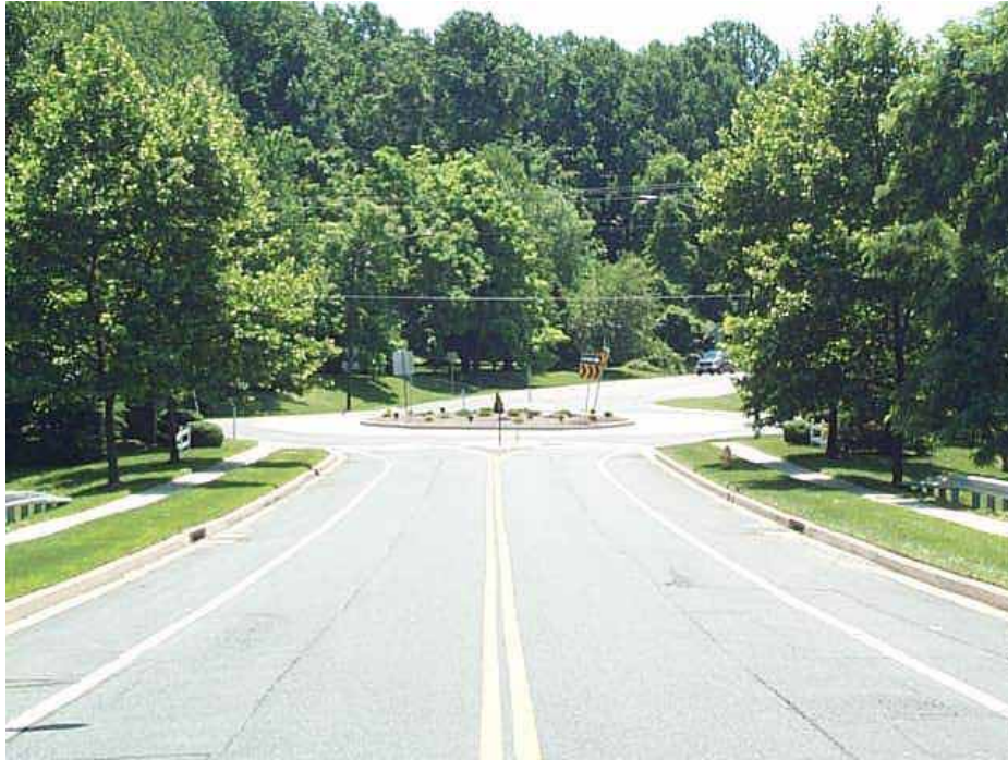
Tollgate Road/Wheel Road Roundabout
