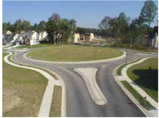
Roundabout currently under construction (Sept. 2004)
