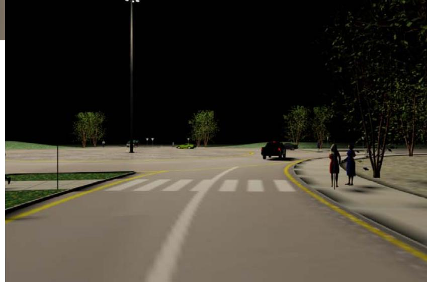
For the roundabout with approach lighting we used 8-10 meter poles with 250 watt high pressure sodium full cutoff cobra head luminaries.
