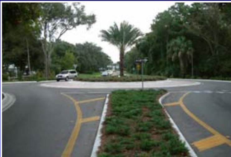
Good drivers can pass through a 23 mph designed roundabout at 27 mph and more than 30 mph through a roundabout with 25 mph design speed. I prefer to limit all of my roundabouts to 23 mph or less to truly limit vehicle speeds and reduce the lowest crash rates
