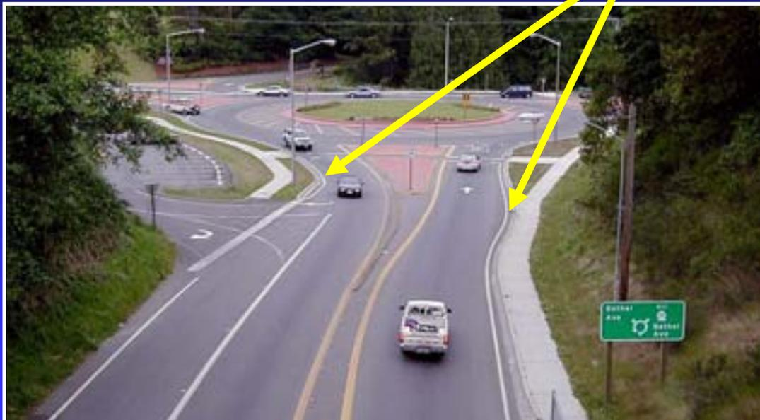
See how kinks, even in the pavement markings, degrade the overall appearance of the roundabout
