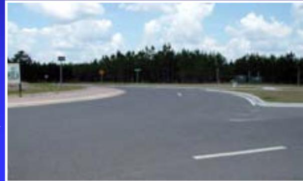
Two Lanes Merge into one within a roundabout from both left and right create a free-for-all that forces drivers to merge while traveling a double reverse curve
