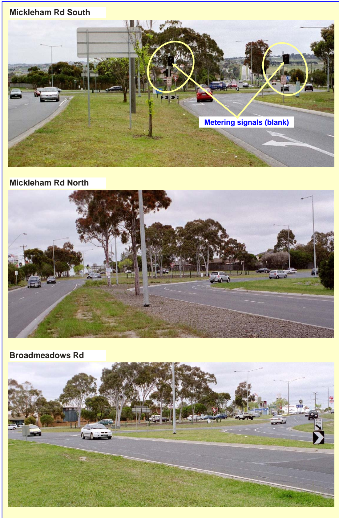
Figure 7 - Mickleham Rd and Broadmeadows Rd Roundabout, Melbourne, Australia (all photos and drawings in this paper are modified to show driving on the right-hand side of the road)
