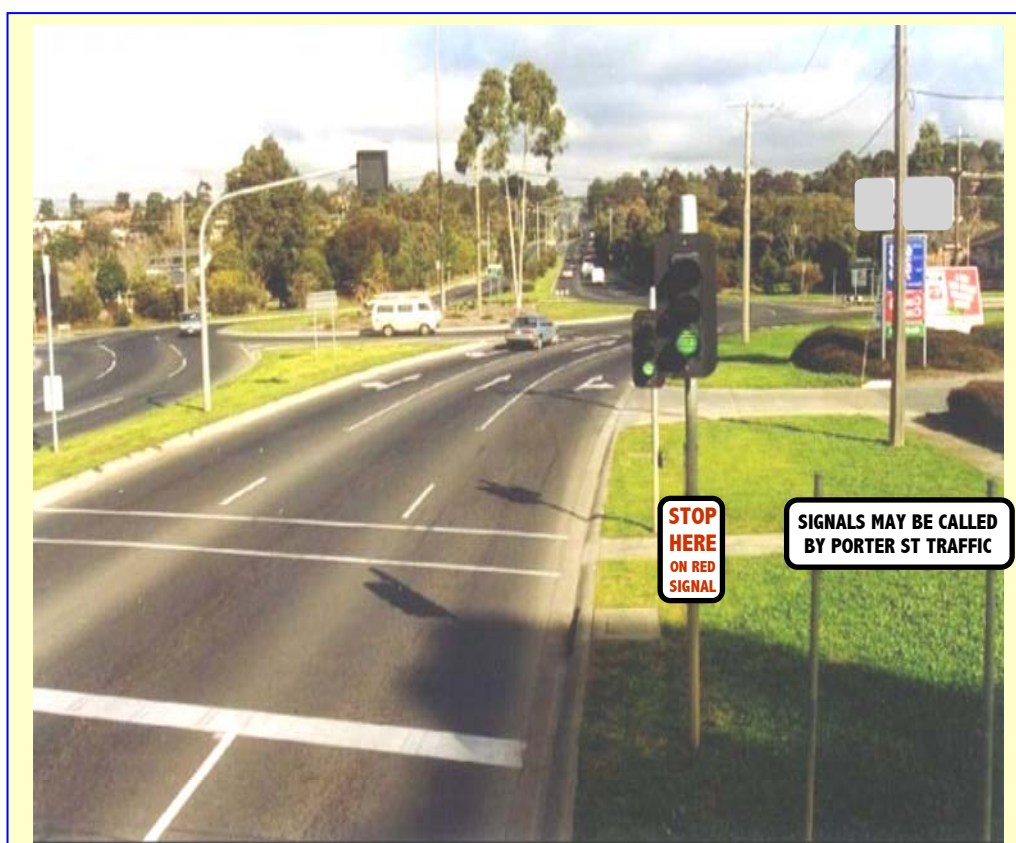
Figure 5 - Use of pedestrian-actuated signals for roundabout metering at Fitzsimons Lane - Porter St Roundabout, Melbourne, Australia (photo modified to show driving on the right-hand side of the road)
