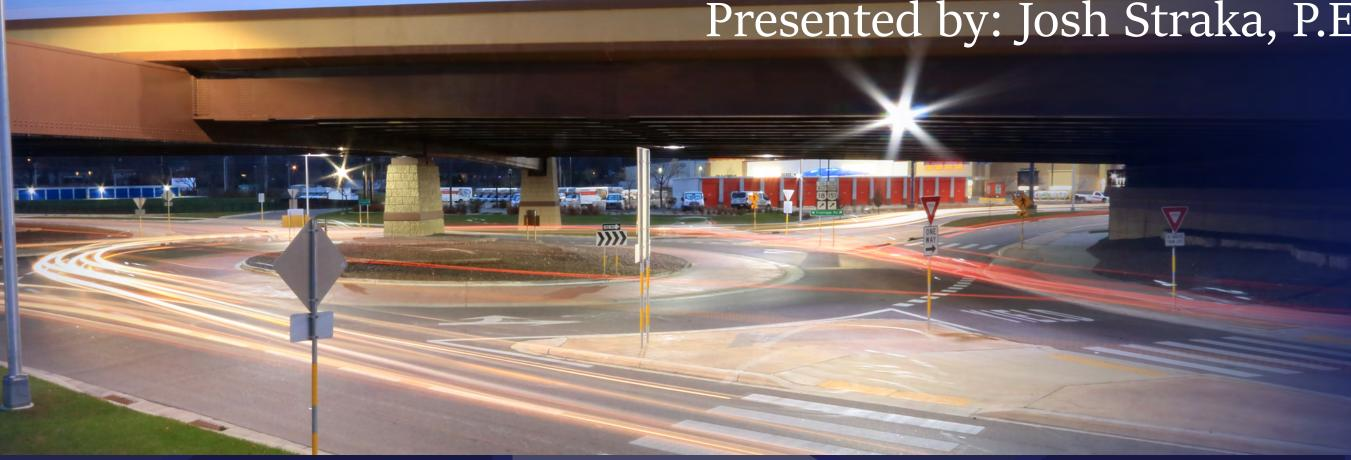
The U.S. Highway 18/151 (Verona Road) project reconstructed one of the busiest corridors and interchanges in Madison, Wisconsin, and includes an unprecedented approach to roundabout installation. Completed in 2016, Stage 1 of 2 cost approximately \$100 million, which included construction of 3 new major structures all within less than 1 mile: a single-point interchange (SPUI), a jug-handle-style intersection, and a roundabout directly underneath Verona Road.
