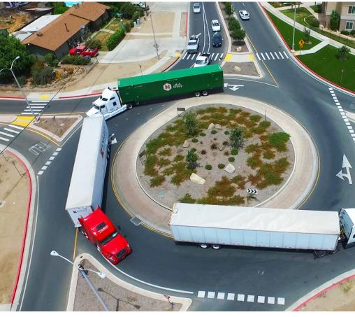
designed to accommodate 18% 5-axle trucks, which equates to over 400 trucks entering and/or leaving each and every day. The construction was staged to accommodate truck access 24 hours a day, 7 days a week. The roundabout was constructed with minimal delays to the distribution center traffic.
