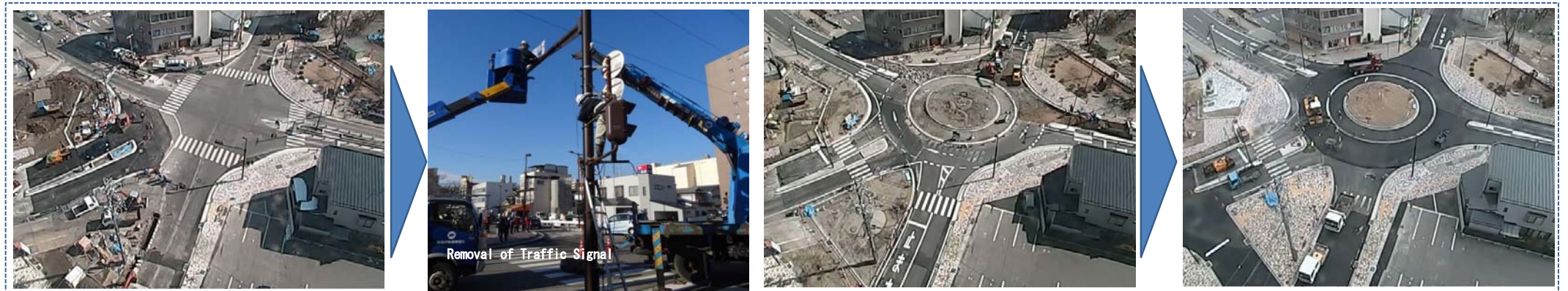
Photo-3 Transformation from signalized to roundabout intersections
