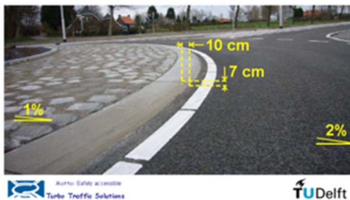
Figure 12. Low truck aprons in the Netherlands (Top-source LGH Bertus Fortuijn) and the UK (Bottom- Source: Clive Sawyers 2012)
