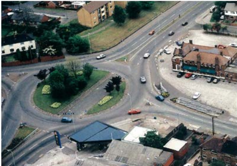
Figure 15. Roundabout showing straight-through path for large vehicles (Source: K-State Roundabout sent by L.G.H. (Bertus) Fortuijn. 2012)
