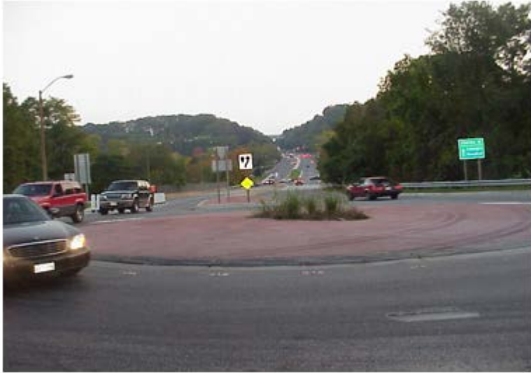
Figure 10. Roundabout north of Baltimore - almost all truck apron (photo by Gene Russell, 2000)
