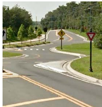
Figure 1 - Not white curb extension added post construction to slow vehicles
