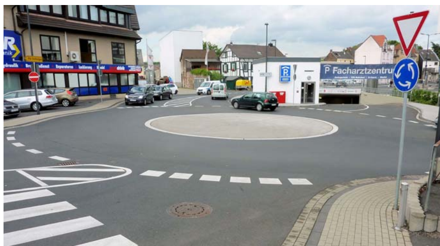
Figure 4 : Critical design for a Mini-Roundabout: The central island built of concrete is on the same level as the circular lane (lack of a delta of 4 – 6 cm). This reduces the acceptance of a correct driving on the circular lane. The direct access from the circle to private parking positions (left side) gives reason for several conflicts.
