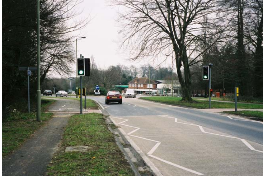
Figure 3: Signal controlled crossing close to a roundabout
