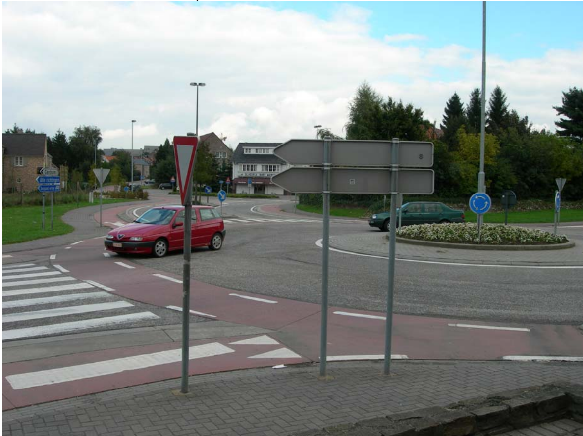
Picture 1 – Roundabout with cycle lanes
