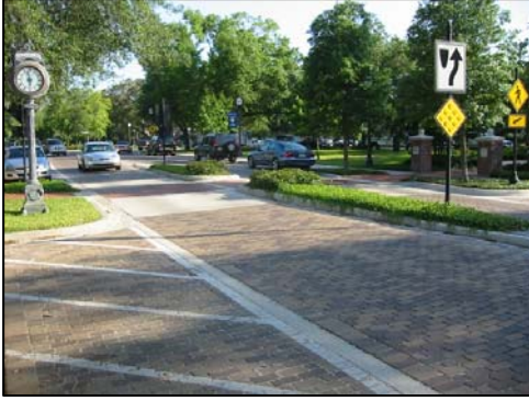
The raised midblock pedestrian crossing located between the two roundabouts
