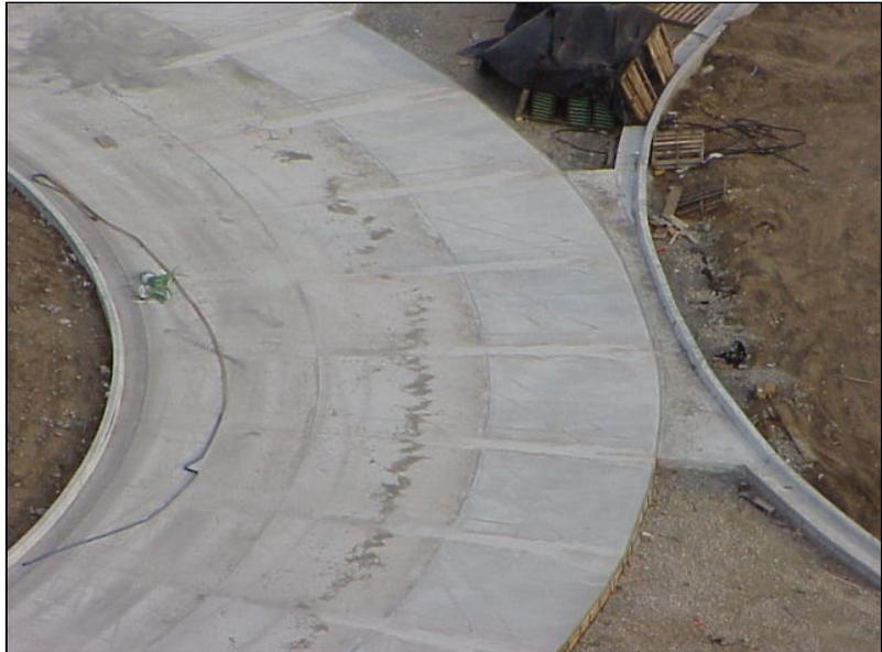
Figure 7: Sections of the curb were placed monolithically with the pavement around curb returns and splitter islands to control cracking and to eliminate small, irregular shaped panels. Note how the contraction joints lined up across the circulating lanes.
