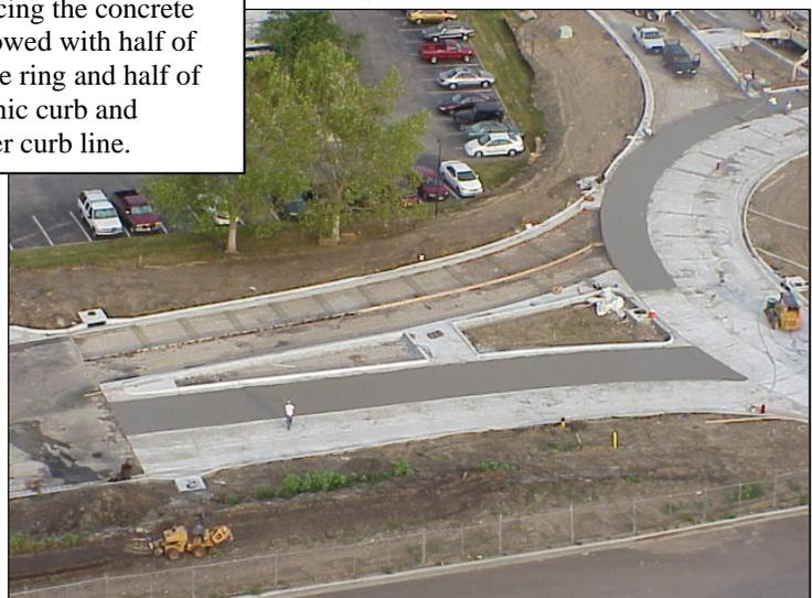
Figure 6: Placement of the concrete in the remaining half of the outside ring of the circulating lanes occurred simultaneously with some of the approach and departure lanes. The concrete pavement ended at the end of the splitter island. The pavement approaching the roundabout was asphalt, except on the east leg which was totally concrete.
