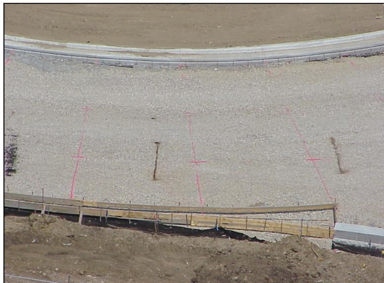
Figure 4: Construction joints on the curb of the internal island needed to align with the construction joints on the outside curb line to avoid reflective cracking across the circulating lanes. There were many control points that needed to be taken into consideration and the painted joint pattern on the aggregate base provided the proper guidance.
