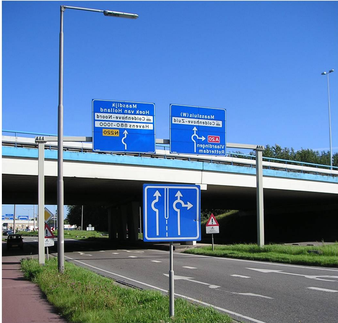
FIGURE 11 Road Signs to assist entry lanes at roundabouts in The Netherlands (note: image is reversed)
