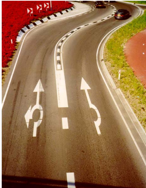
FIGURE 5 Lane Use Arrows in The Netherlands (counter-clockwise traffic)
