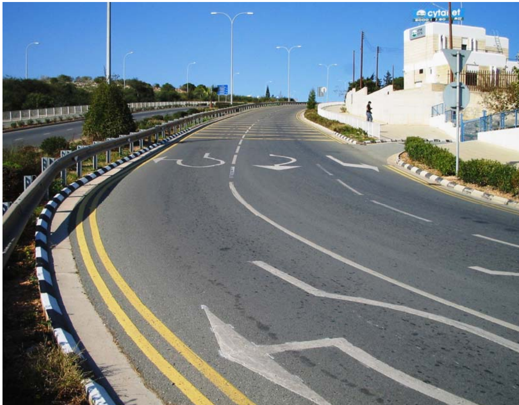
FIGURE 9 Lane Arrows at Ayia Napa Roundabout in Cyprus (Photos) (clockwise traffic)
